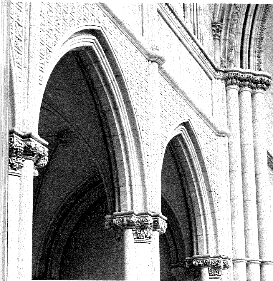
49 Mr Godfrey's work can be seen on the cluster columns at the entrance to the sanctuary and the carved capitals on all the columns on both sides of the nave. On twelve columns the carvings in Oamaru stone encircle the whole column. Although Mr Godfrey uses an endless variety of carvings — flowers, petals, birds, figs, grapes, leaves, lizards, petals and ferns — no two capitals are alike or the carving repeated. Carved into the Oamaru stone wall above and between the arches are examples of Mr Godfrey's carving in oak leaf. See Photo No. 42.
