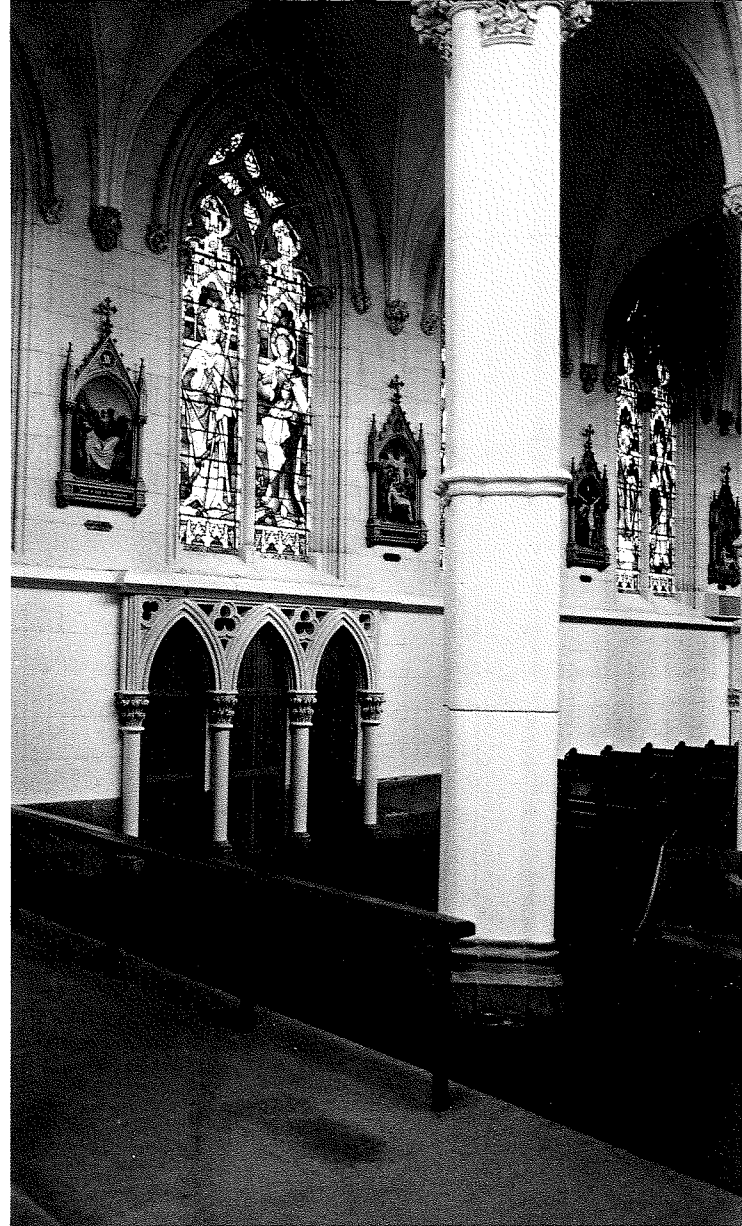
46 The three confessionals were built by Parker and McNamara in bluestone between the lower buttresses on the north wall. The arches are beautifully made and the stone carving at the top of the columns is that of Mr Godfrey. The carving designs are different on each column.
