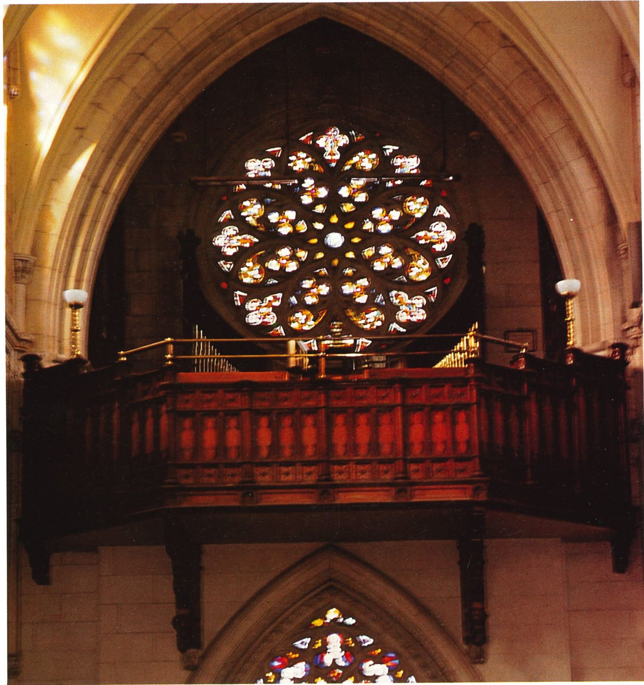
72 In December 1883 Mr D. W. Woods, the contractor for the carpentry and joinery in the Cathedral, began the preliminary work of the choir gallery. In 1897 it was decided that the choir gallery had been placed too high, and to remedy this defect and improve the choral acoustics Mr Woods was asked to lower the gallery by two feet. At the same time, it was decided to extend the gallery further out into the nave to provide additional accommodation. A feature of the gallery is the rich paneled and carved balustrade at the front in a semi-circular form. The timbers used were Kauri for the lighter colours and imported Cedar for the darker colours.
